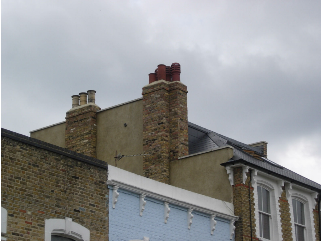
Figure 7: Roof extension viewed from the north
