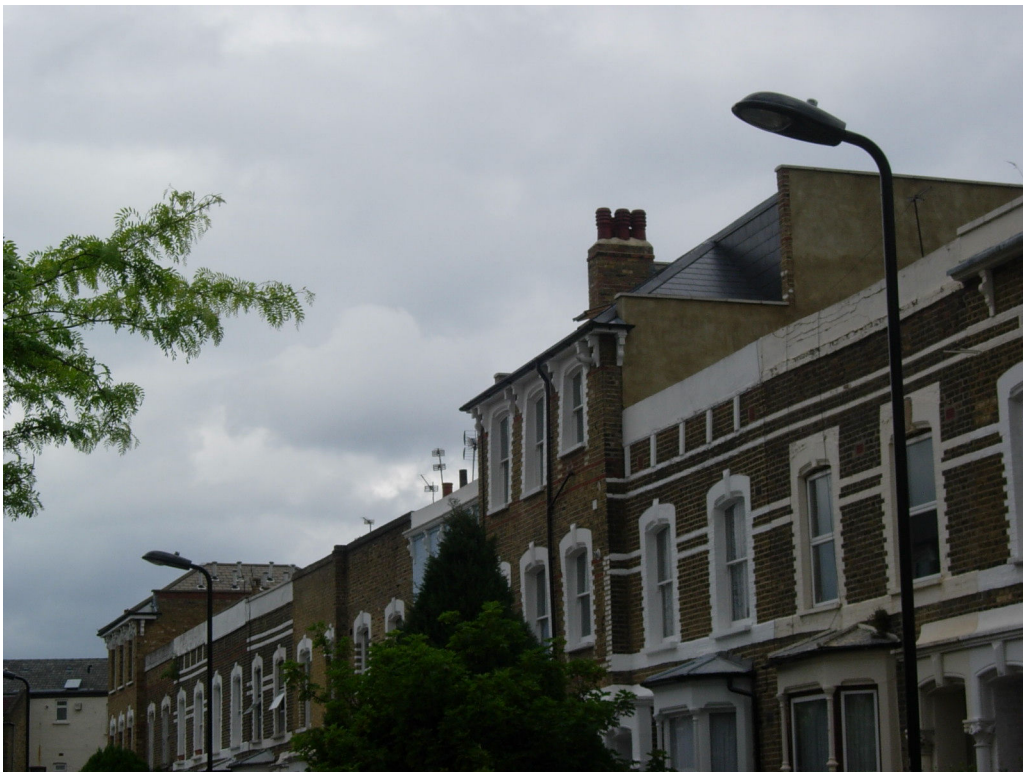
Figure 8: Roof extension viewed from the south
